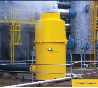
For pre-commissioning, a FourQuest Energy designed continuous low-pressure steam blow technique is the leading accepted practice for cleaning steam system circuits.
