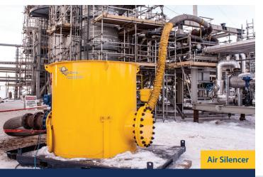
Engineered air blowing is a predictable method to remove construction debris, loose rust, liquids, and other contaminants from process piping.
