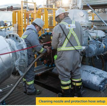
Hydro-milling, also known as water jetting, retro-jetting or hydro-jetting, is an efficient method of cleaning industrial piping through the implementation of high-pressure water nozzles and jets.
