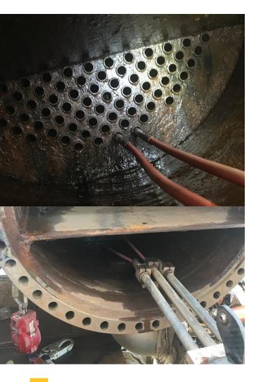
Fouling components and rust gradually form during operational processes that will eventually require removal. Our high-pressure washing equipment is designed for various industrial applications that will leave equipment surfaces free of deposits and rust.
