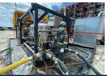
FourQuest Energy utilizes proven proprietary flushing skids (FS), which are self-contained, self-sufficient units that include an onboard pump, heater, mixing tank, reverse flow manifold, and filtration system to capture insoluble matter.
